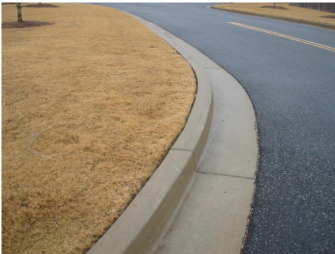
Example of concrete curbing
