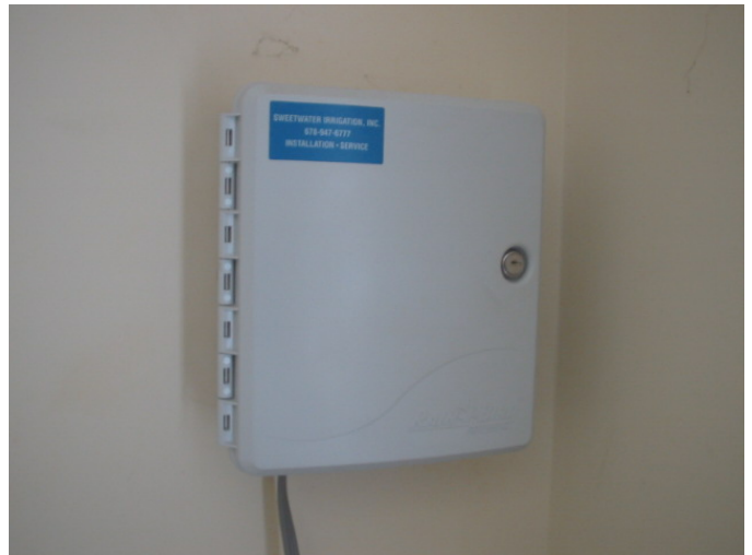
Example of irrigation control board (1 of 2)
