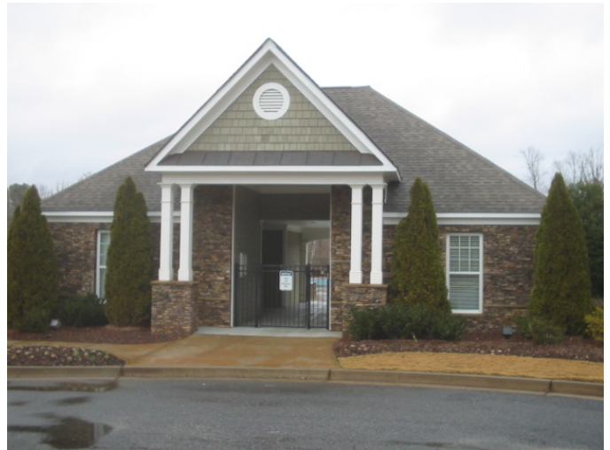
Poolhouse front elevation. Note stone veneer and shingle siding at gable, windows.
