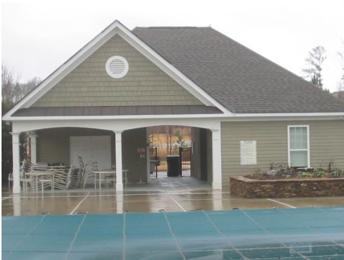
Poolhouse rear elevation. Note siding materials, metal roofing on eave return, window
