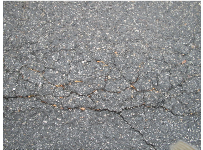
Example of asphalt alligating near poolhouse
