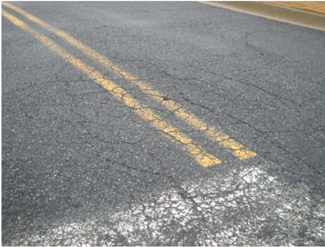
Example of asphalt alligating at amenity entry
